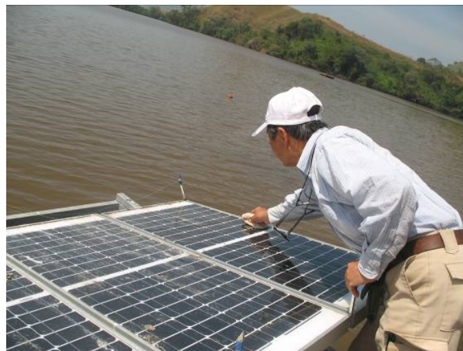
Figure 7: Cleaning of the solar panels
